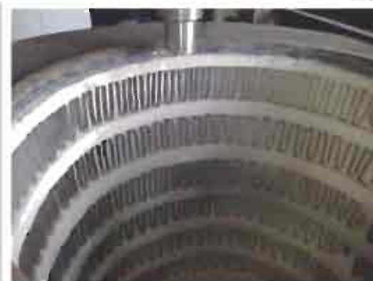
LINING OF LPDC FURNACE
